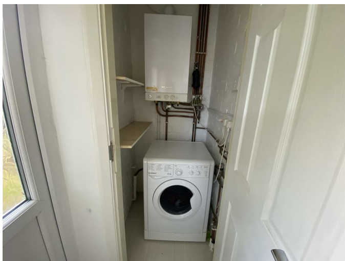
Utility Cupboard 4'2 x 3'3 (1.27m x 0.99m)
